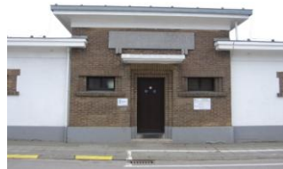
Station de pompage
